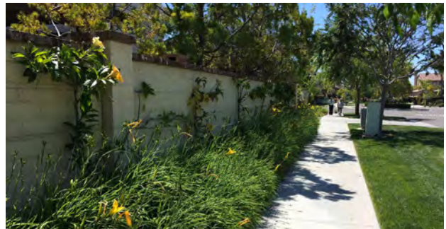
Masonry Community Wall
